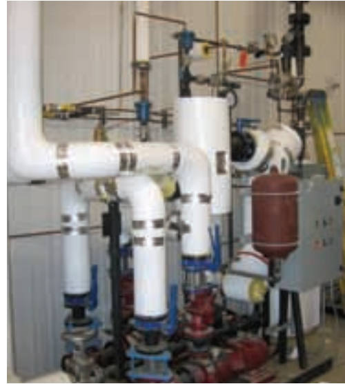
Building Heat: 175 US gpm Glycol ; 55° F → 95 ° F Back pressure 10 psig ; steam @ 110 psig Floor space 4' x 6' x 7' H c/w circulating pumps, expansion tank, air separator, control panel
